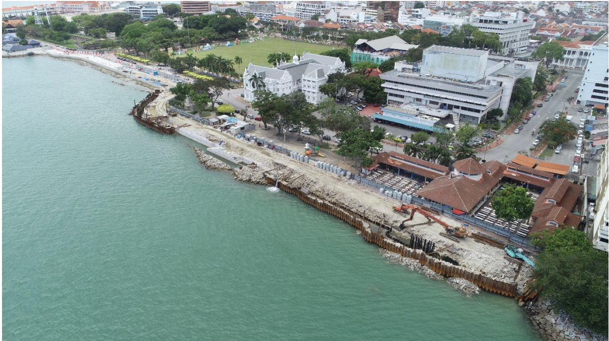
Seawall Upgrading: Under construction
