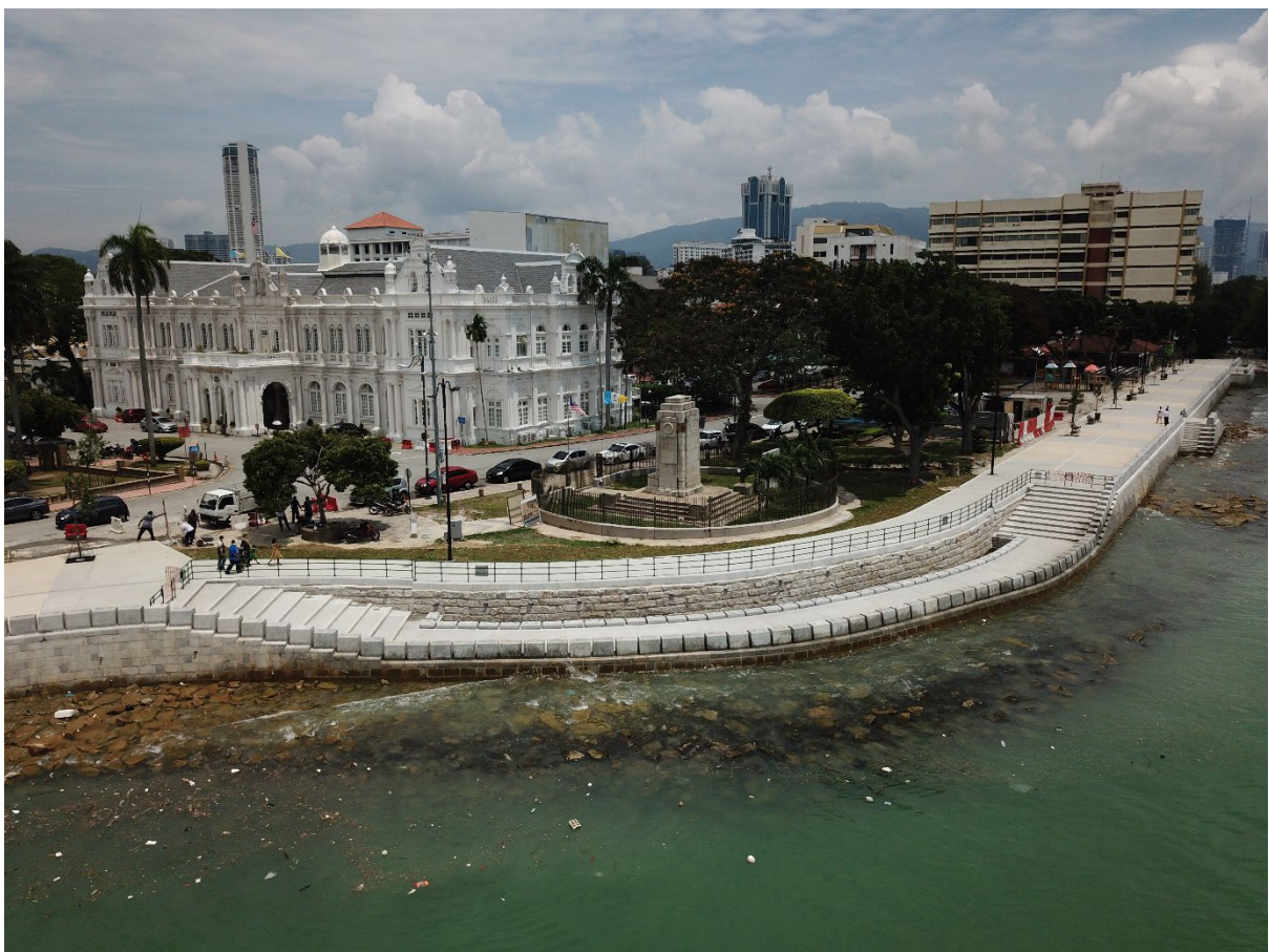
Completed Seawall Upgrading & Promenade
