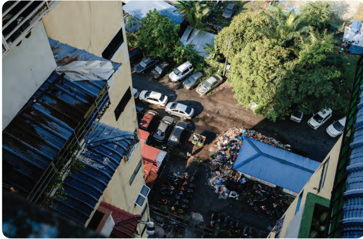
Overflowing rubbish around the garbage disposal room is a common view from the apartment windows.
