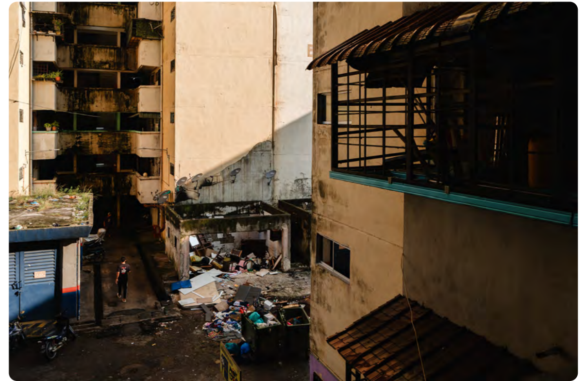
A solid waste disposal facility suffering from acute neglect.
