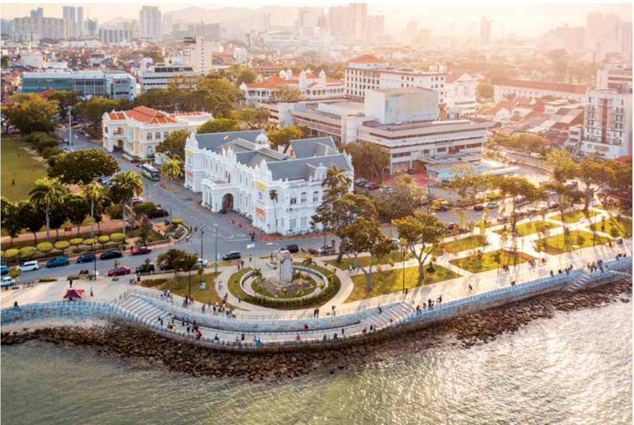
The expanse of the Linear Garden with the Cenotaph rotunda and the two-tiered seawall promenade below.
