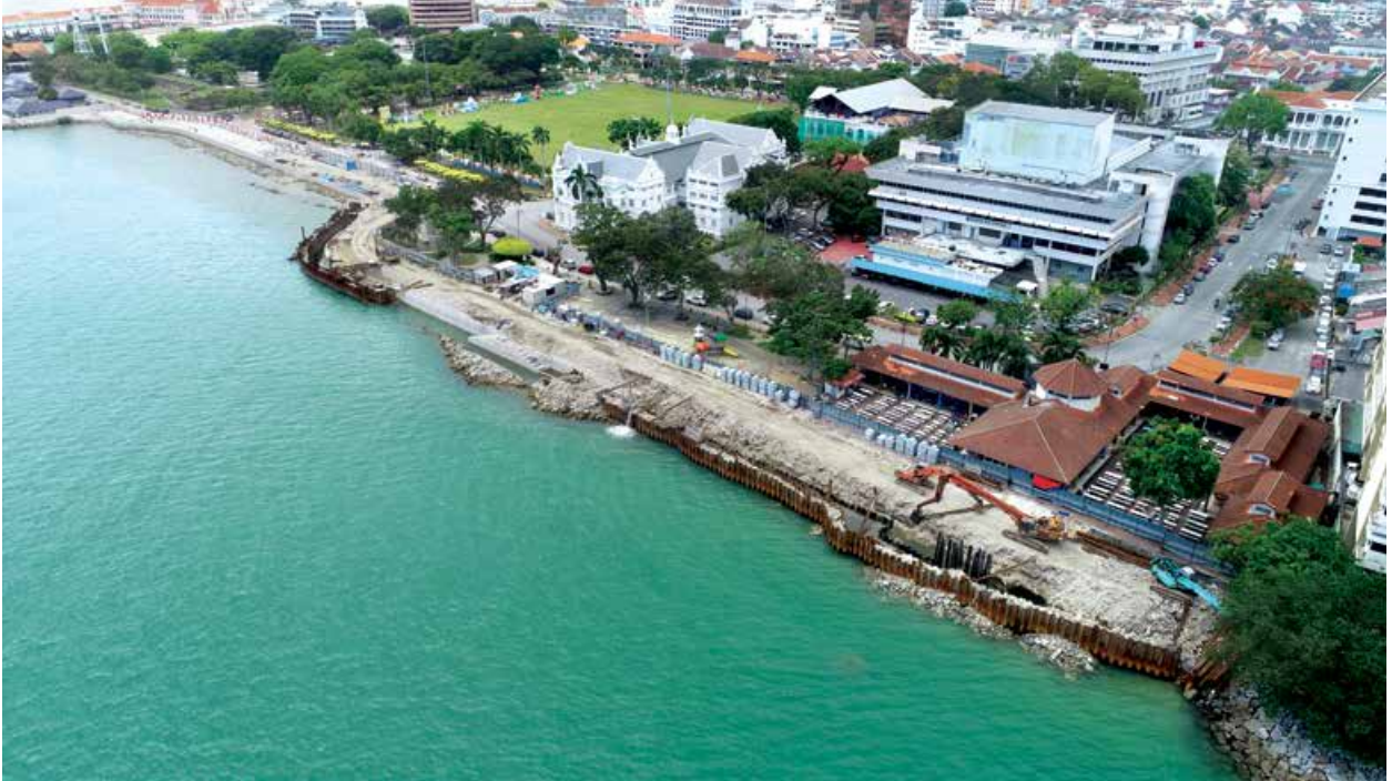
Seawall and Public Seafront Promenade under construction.
