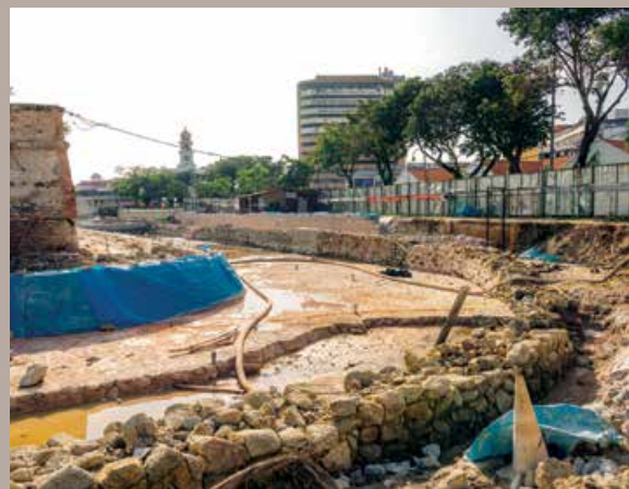
Modular sub-base under construction (left) and layered paving of the water basin (right).
