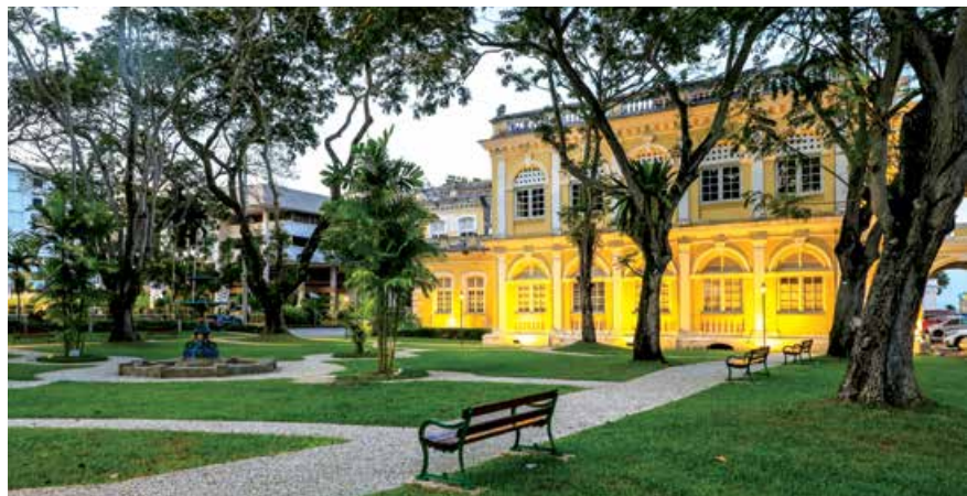
The Fountain Garden after restoration.
