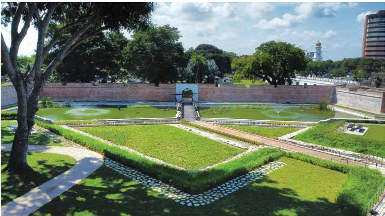
West moat after completion.
