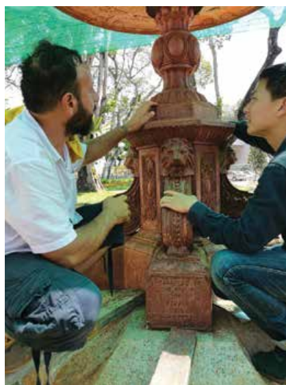
The cast iron fountain under restoration.
