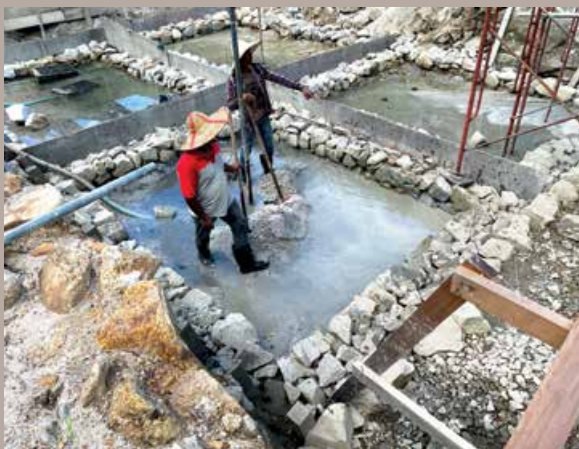
Modular sub-base under construction (left) and layered paving of the water basin (right).
