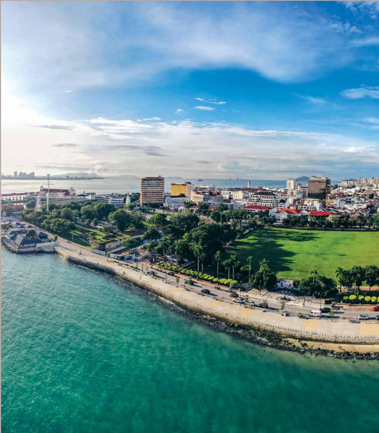
Completed Seawall and Public Promenade upgrading with the Cenotaph in the foreground and green expanse of the Esplanade behind.
