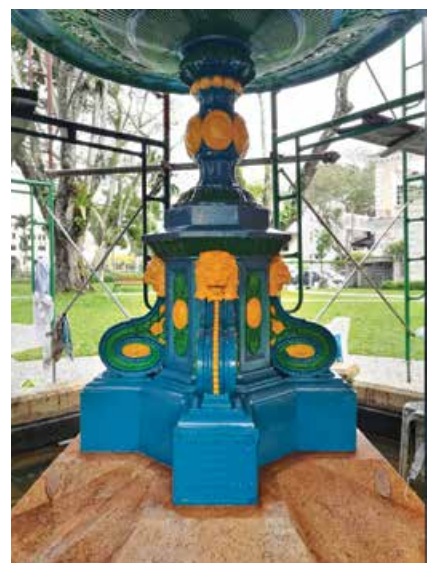
The original paint layers applied during the Victorian period were identified and reinstated.
