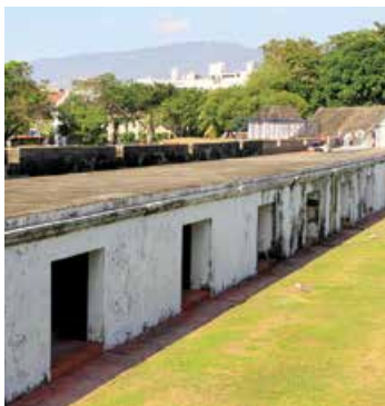
Storage Rooms before intervention.
