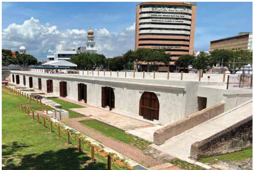
Restored Storage Rooms.
