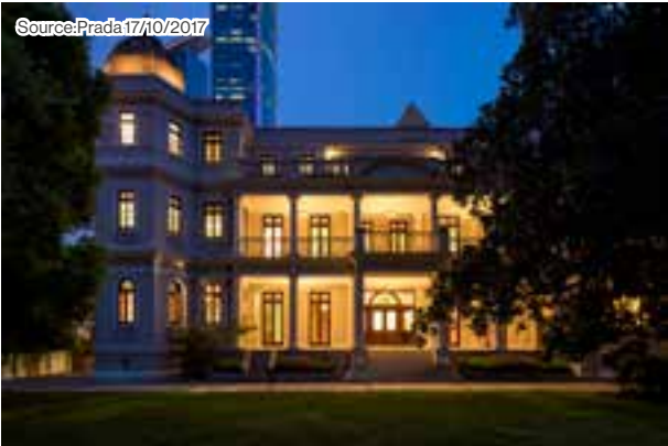
Prada Rong Zhai, a restored early 20th century mansion in central Shanghai.
