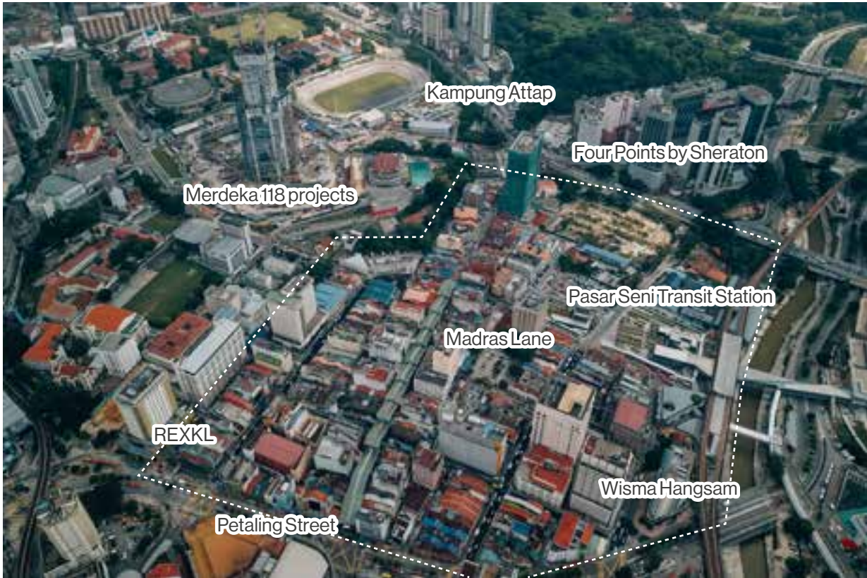
Aerial view of the Petaling Street Precinct, 2018
