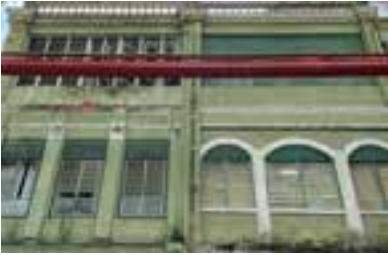
4 Shophouses at Jalan Petaling
