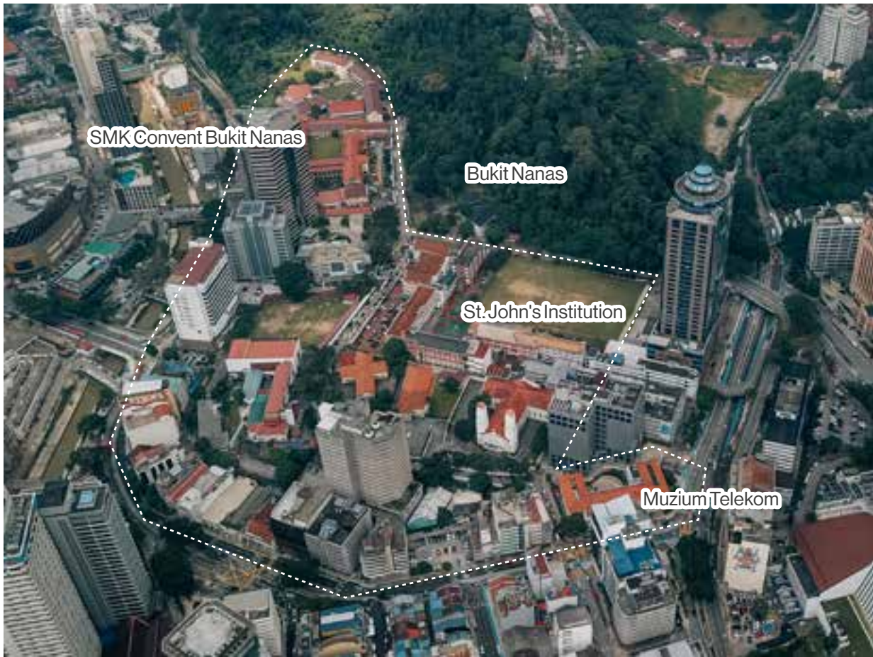
Figure 1.20: Aerial view of the Education Precinct, 2018
