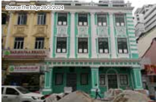
Lebu Ampang shophouse restored by Think City in collaboration with DBKL and CGB Consultants (Ar. Junn Ng, Conservation Architect).
