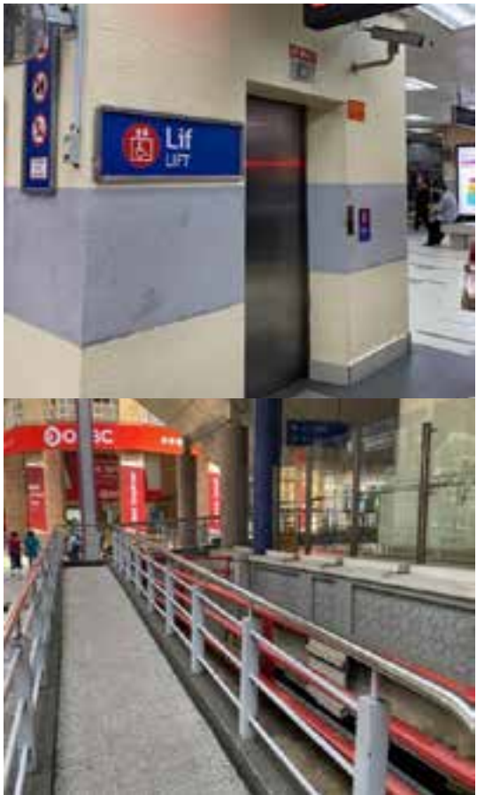
Figure 4.28: Lift (top) and accessibility ramp (bottom) at Masjid Jamek LRT station
