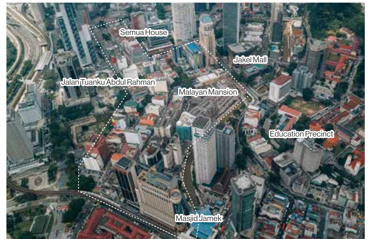
Aerial view of the Traditional Shopping Street Precinct, 2018
