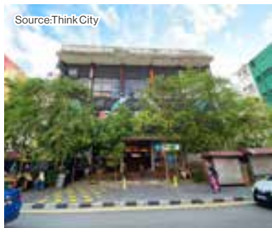
REX KL, restored from an old cinema—now offers a theatre, event space and retail. This project was executed by a group of creative entrepreneurs led by Shin Tseng and Shin Chang.
