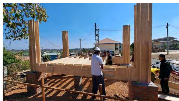
Figure 5(f). Shelter construction in Taung Gyi township.
