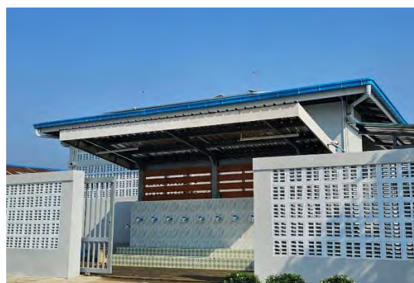
Figure 5(e). Solar powered Standalone water treatment station.
