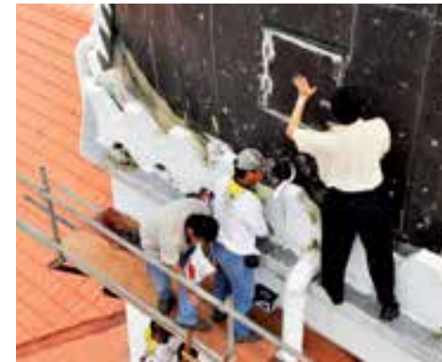
Copper cladding on the dome of the Masjid Kapitan Keling.
