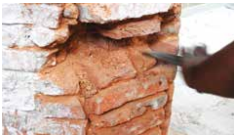
Cleaning out the old mortar to ensure the new mortar can bond to the bricks.
