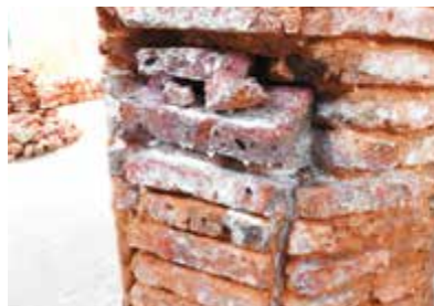
Finding brick pieces that fit into the empty spaces, and checking for size and alignment.
