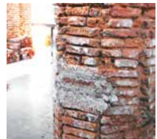
Deep areas are filled in with small broken brick pieces and lime mortar, and allowed to dry slowly, spraying with lime water every few days.
